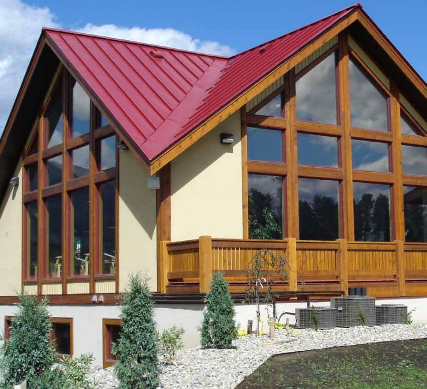
Northern Development's first project investment, the Valemount Visitor Information Centre is a 3,600 sq ft facility focused on promoting local and regional tourism while also including new municipal offices.
